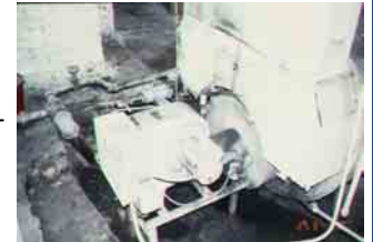
Old steel boiler retrofitted to a new high efficiency steam boiler
